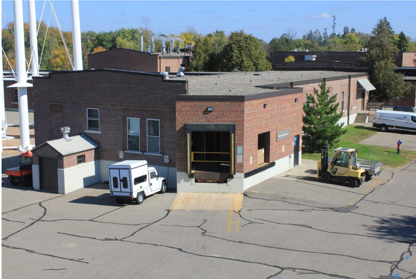
Building 14 (1924): This one story building serves as the primary warehouse.
