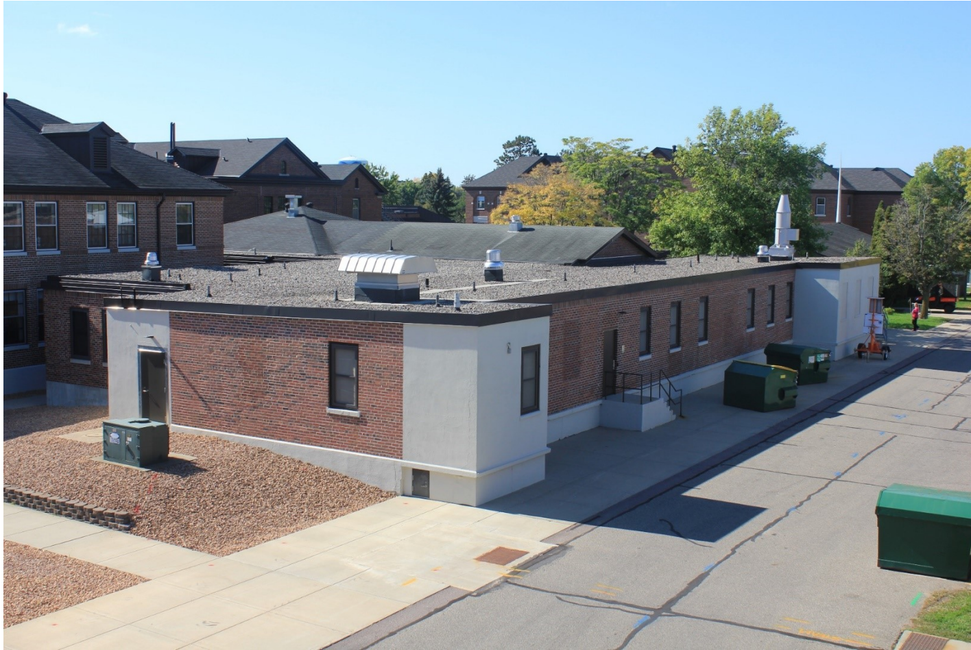
Building 5 (1923): This one story building houses the Pharmacy.
