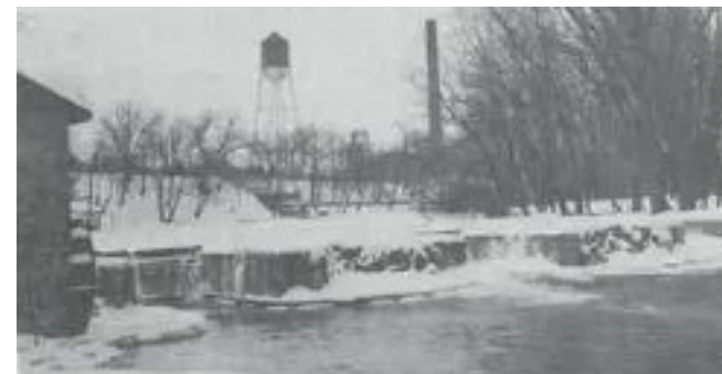
The granite scrap damn in the Sauk River. The reservoir behind the dam was used to form a smooth ice field from which sufficient ice was harvest in the winter to keep all summer in the station's cool houses. (1939).
