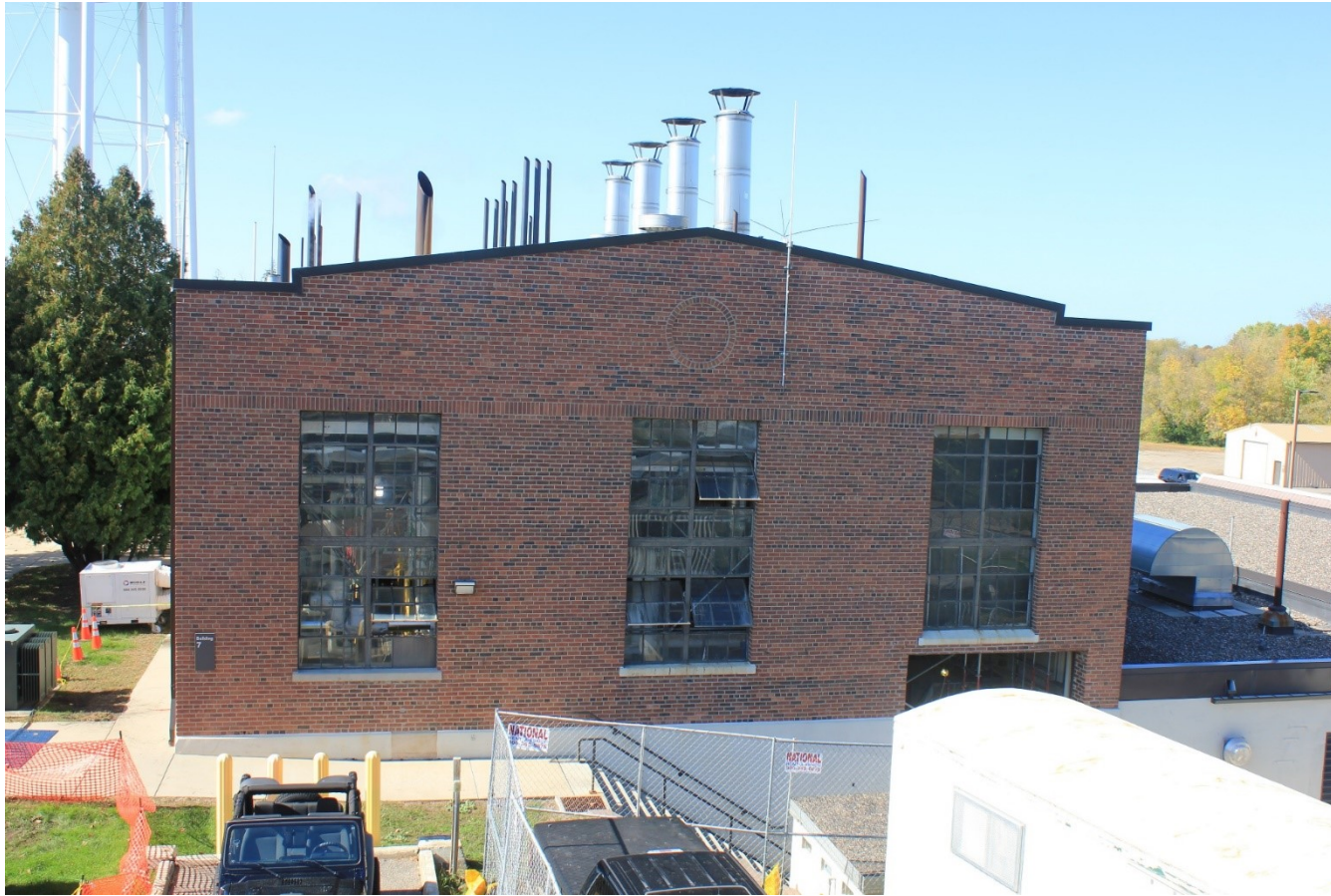
Building 7 (1923): This one story building houses the boiler plant.
