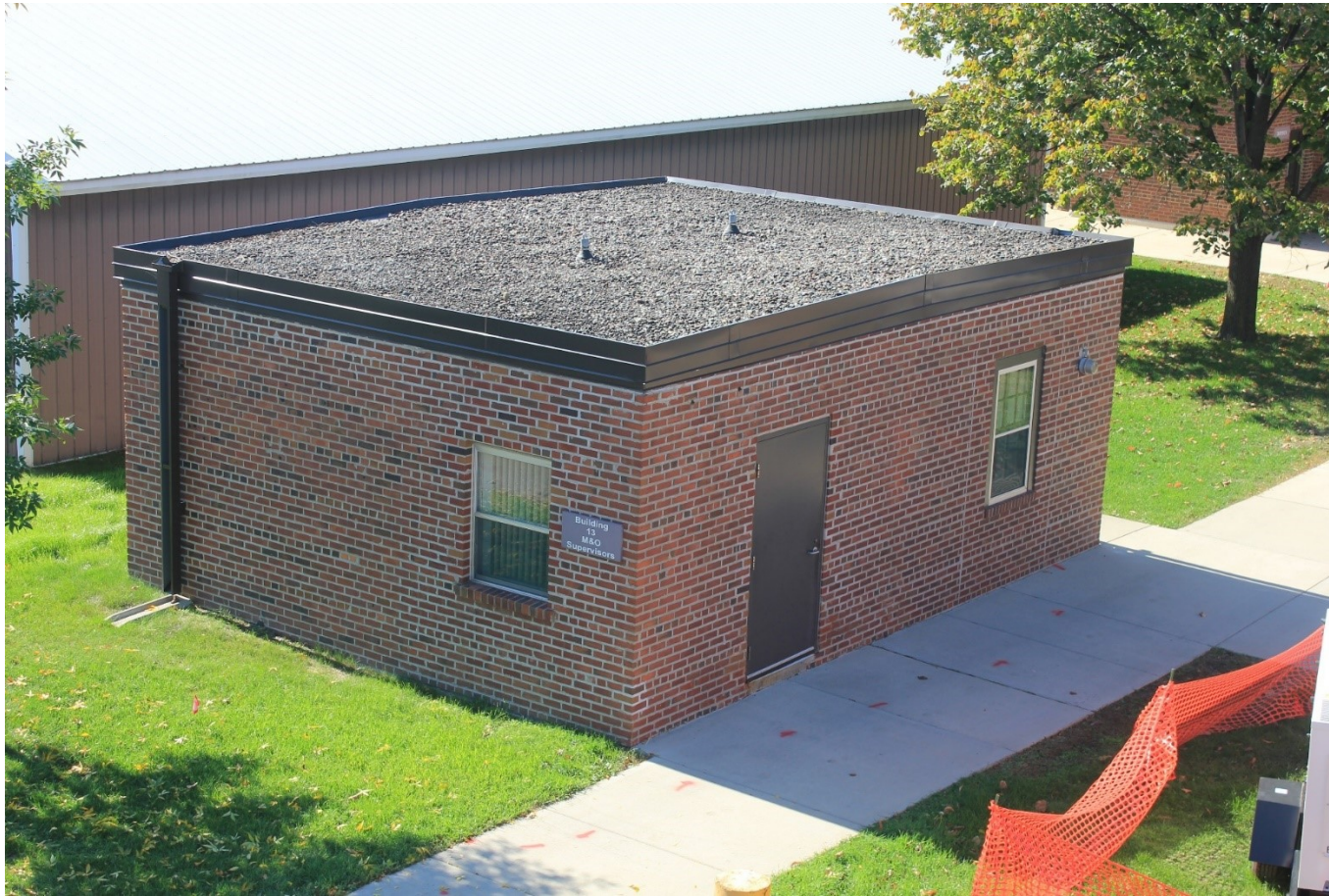
Building 13 (1923): This one story building houses facilities management offices.
