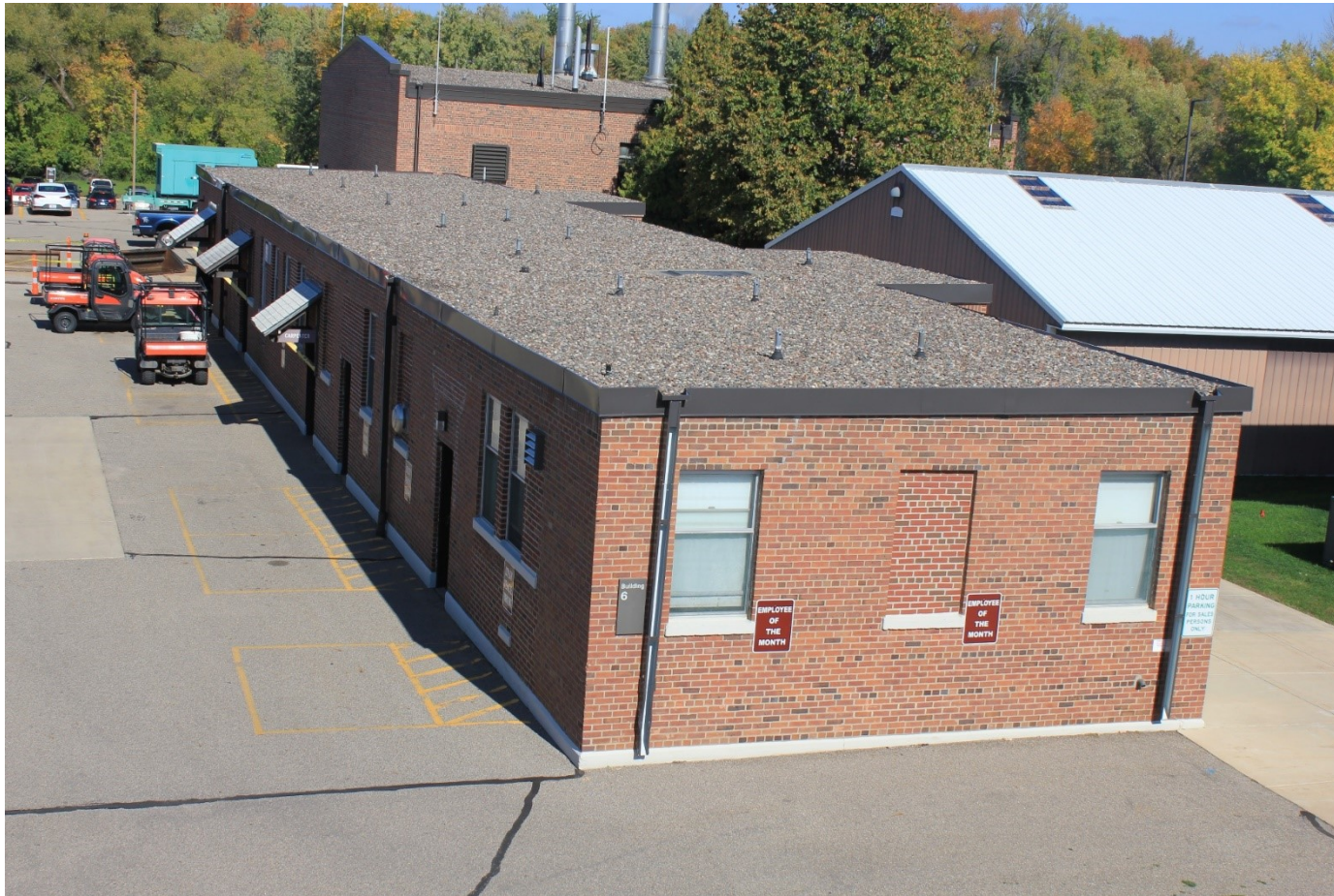
Building 6 (1923): This one story building houses Facilities Management workshops.
