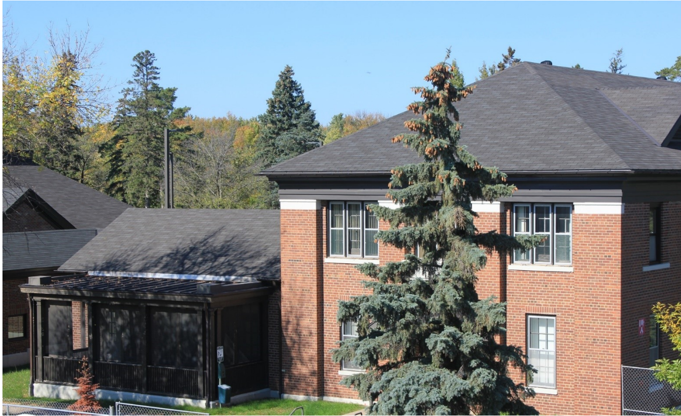
Building 9 (1923): This two story building houses Mental Health service's administrative spaces and the VA Police station.
