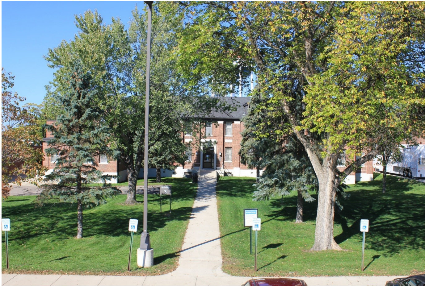
Building 3 (1923): The first floor houses the Dental Clinic and the second floor houses the Facilities Management offices.
