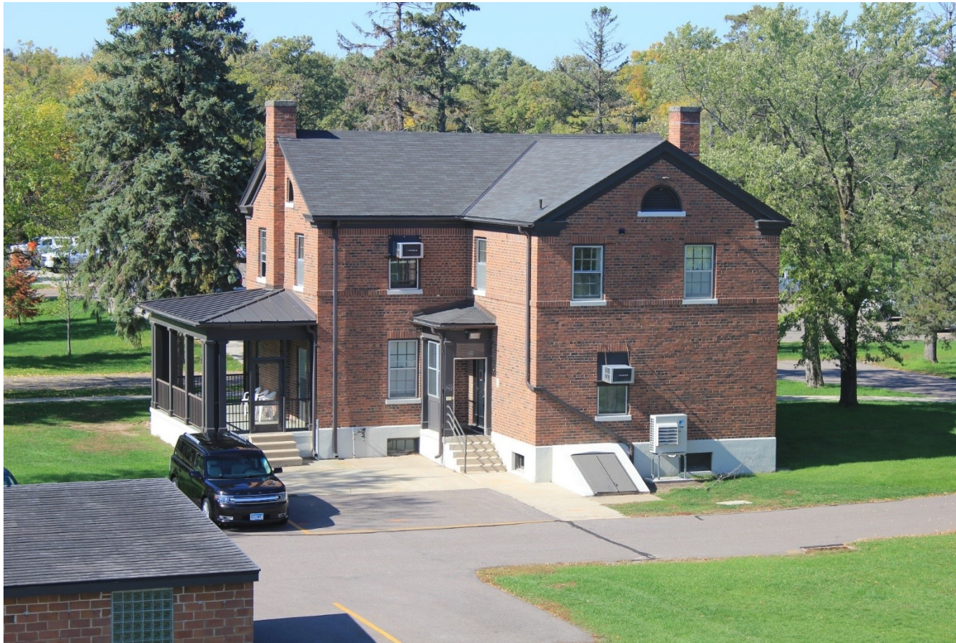
Building 11 (1924): This two story building houses administrative offices.
