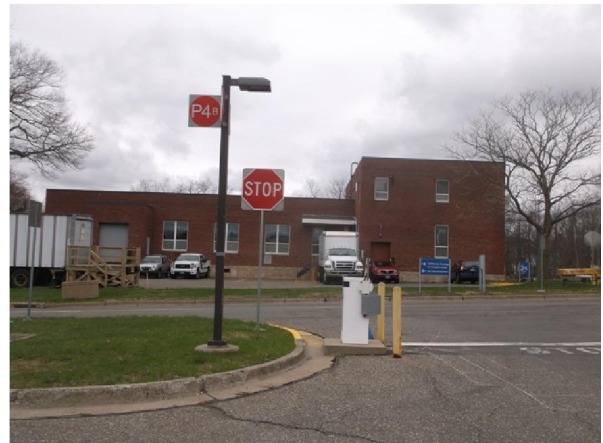
Photo #16: North adjoining Building 24 beyond Ring Road.
