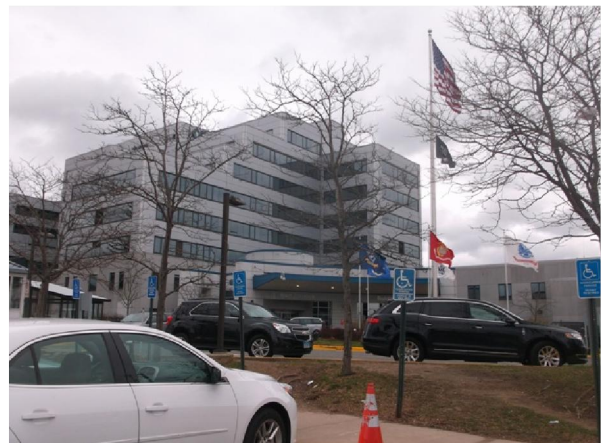
Photo #12: Southeasterly adjoining Building 2 (Main Hospital) beyond the main entrance drive.
