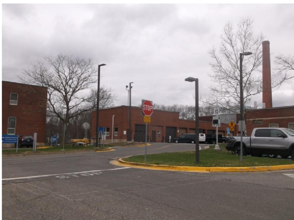
Photo #17: North adjoining Building 22 beyond Ring Road.
