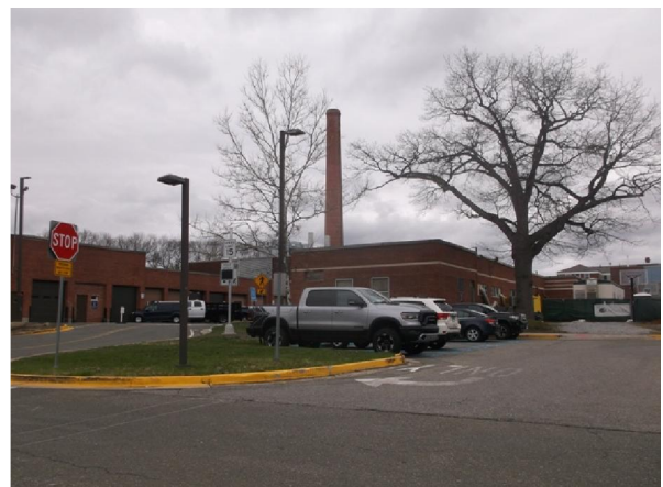
Photo #18: Northeast adjoining Building 21 beyond the main entrance drive.
