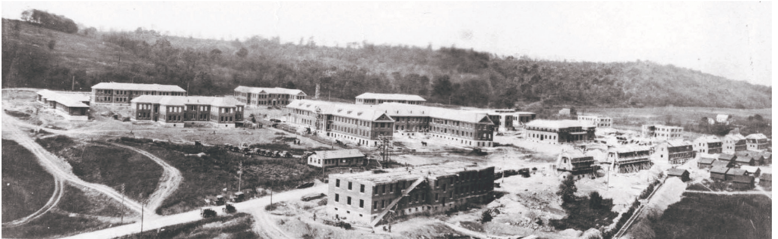
Construction of the Veterans Bureau Hospital, c. 1923 Hathaway Art Studio, Chillicothe, Ohio
