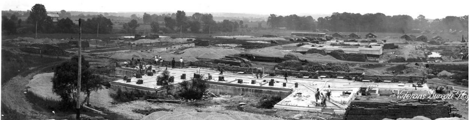
Construction of the Veterans Bureau Hospital, Camp Sherman O., July 3, 1923 No. 14, Hathaway Art Studio, Chillicothe, Ohio
