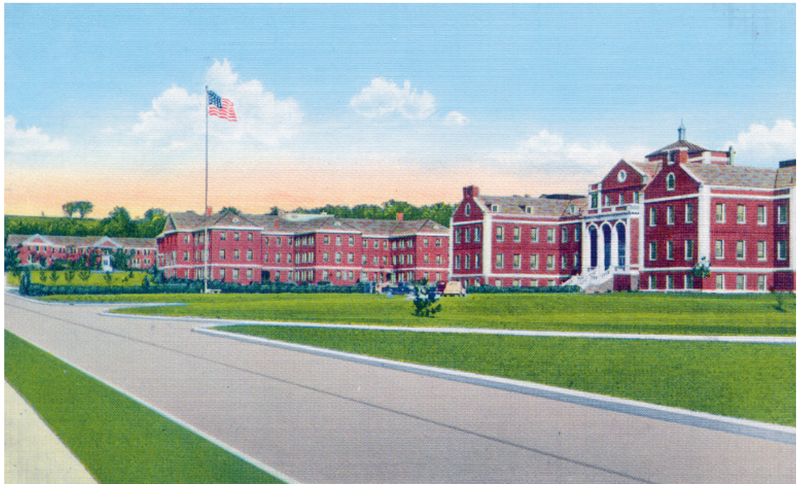
Main Buildings, Veterans Administrative Facility Chillicothe, Ohio
