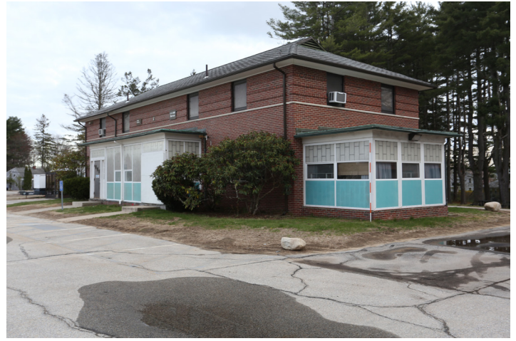
Photo 16: 2022 photograph of one of the Staff Quarters.
