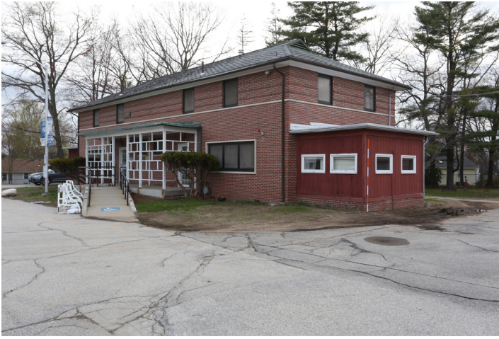
Photo 15: 2022 photograph of one of the Staff Quarters.
