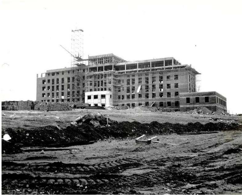
Photo 5: 1949 photograph of the main hospital building under construction.
