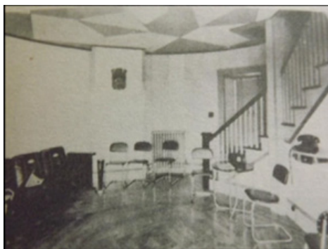
Interior photograph of the ground floor of Smyth Tower.
