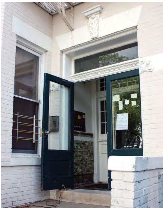
Fig. 16. Historic vestibules retain conditioned air in the living spaces.
