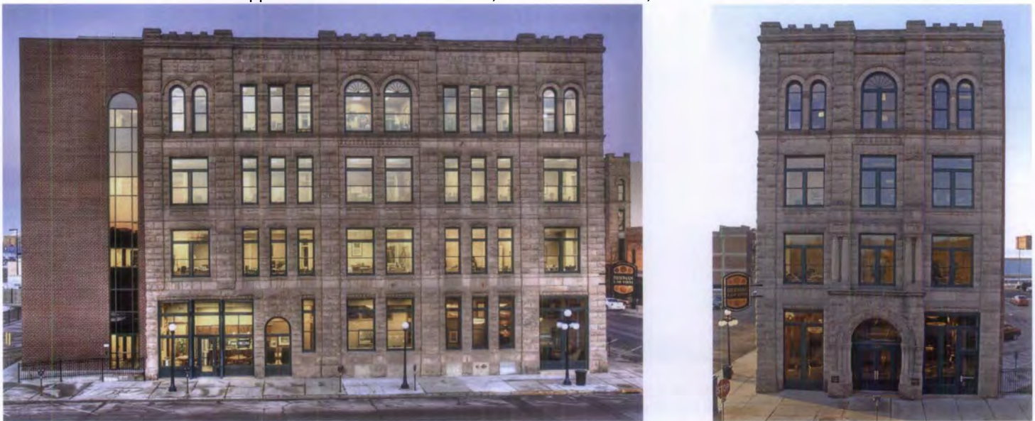
Figure 27. Although the new brick stair/elevator tower (left) is not visible from the front (right), it is on a prominent side elevation of this 1890 stone bank. The compatible addition is set back and does not compete with the historic building. Photos: Chadd Gossmann, Aurora Photography, LLC.
