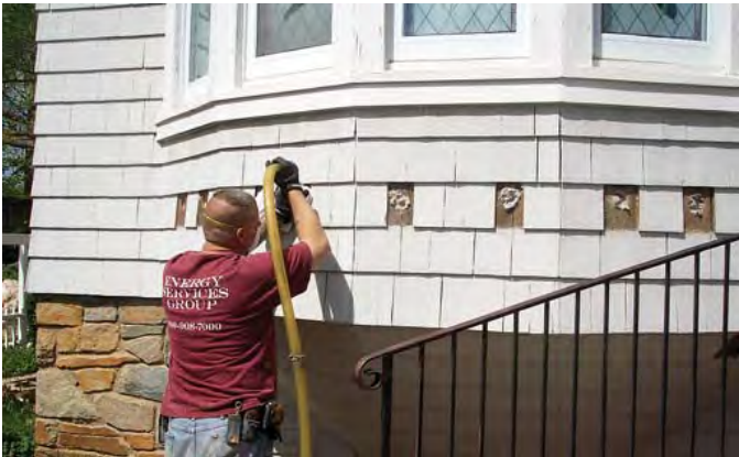
Fig. 18. Dense-packed cellulose insulation is being blown in through holes drilled in the sheathing. Once the operation has been completed, the shingles will be reinstalled. Photo: Edward Minch.
