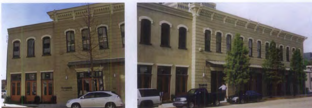
Figure 28. A small addition (left) was constructed when this 1880s train station was converted for office use. The paired doors with transoms and arched windows on the compatible addition reflect, but do not replicate, the historic building (right).
