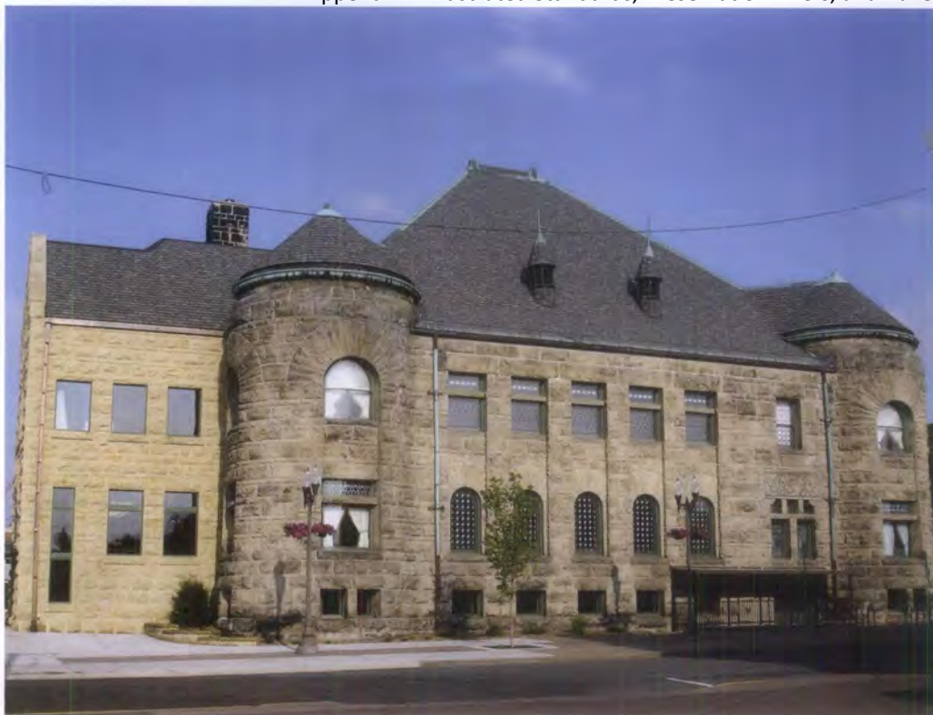
Figure 31. An elevator/stair tower was added at the back of this Richardsonian Romanesque-style theater when it was rehabilitated. Rough-cut stone and simple cut-out openings ensure that the addition is compatible and subordinate to the historic building. Photo: Chuck Liddy, AIA.
