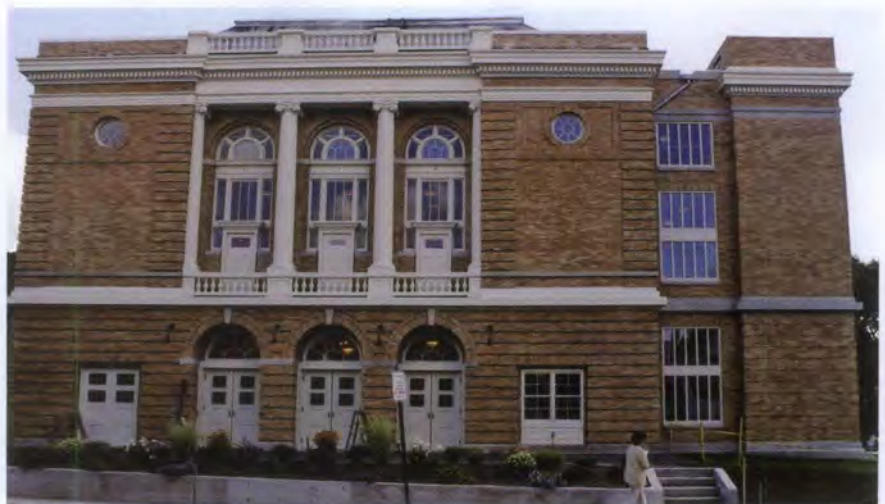
Figure 7. A vacant side lot was the only place a new stair tower could be built when this 1903 theater was rehabilitated as a performing arts center. Constructed with matching materials, the stair tower is set back with a recessed connector and, despite its prominent location, it is clearly subordinate and differentiated from the historic theater.
