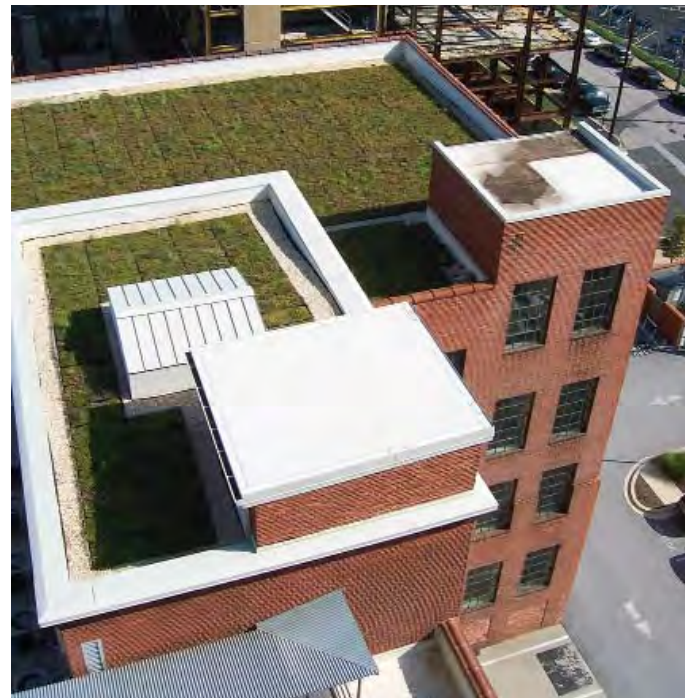
Fig. 22. Installation of both cool and green roofs in an urban environment.
