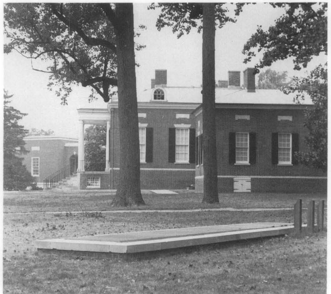
11. During the restoration of this 1806 National Historic Landmark (photo a), a new climate control system was installed. The architects removed all the earlier mechanical equipment from the house and installed new equipment in a 30' × 40' concrete vault located underground 150 feet from the house itself (photo b). Only conditioned air is blown into the house reusing much of the circa 1930s ductwork. Photos: Thomas C. Jester.
