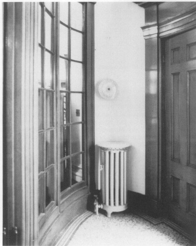
6. A condition assessment during the planning stage would identify this round radiator in a small oval-shaped vestibule as a significant element of the historic heating system. In upgrading the mechanical system, the radiator should be retained. Photo: Michael C. Henry, P.E., AIA.
