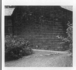
C. The new ground gutter gravel base helps drainage around the concrete foundation (see B above) which is not visible behind the replaced wooden wall shingles. Photo: WPTC, NPS.
