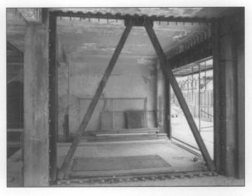
7. More extensive seismic issues can be addressed through structural reinforcement, the most common methods using anchor ties and braces. Shown here is an interior diagonal frame, to be covered, which will dampen and transfer seismic loads in a designed path from foundation to roof. Photo: David Look.
