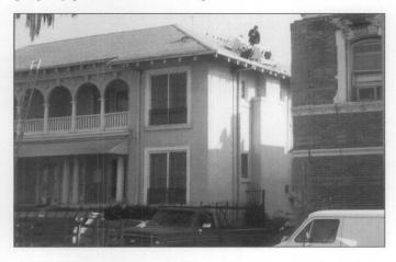
4. The compact size and good condition of the masonry building on the left withstood the earthquake except for the loss of the unsupported chimney at the roof line. The brick building on the right appears to have sustained more damage. Photo: Steade Craigo.
