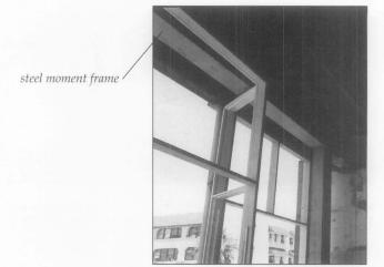
14. The use of a steel moment frame to support the large open storefront during a rehabilitation eliminated the need to place diagonal braces or other intrusive supports in a highly visible area of a historic building. Photo: David Look.
