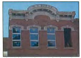
After rehabilitation, the new windows have a threepart configuration that is inappropriate to the historic style of the building.
