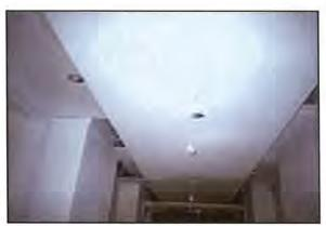
A partial ceiling can cover new systems in a corridor without obscuring existing historic features.
