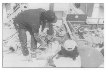
19. A system of core drilling, shown here, removes internal cored sections of unreinforced masonry from roof to foundations and fills them with grout and reinforcing rods. This may be an option for some unreinforced masonry buildings with significant interiors and exteriors, although it is a less reversible treatment than traditional diagonal frames or shear walls. Photo: David Look.
