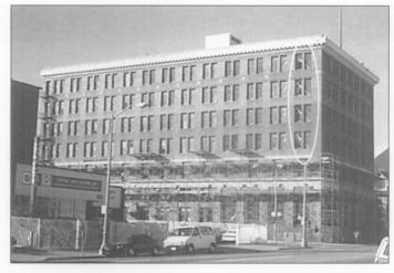
13. Installing diagonal frames, underway in this rehabilitation, are a traditional method of seismic reinforcement. To reduce the impact of the X, K, or diagonal braces, they should be on the inside of the perimeter wall, designed to cross behind solid walls as much as possible, and painted a receding color where visible. Photo: David Look.
