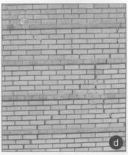
3. Forces from moderate to serious earthquakes caused a) the untied gable to fail, b) the first floor to collapse c) cracks from the pounding effect of adjacent buildings, and d) and diagonal cracks in exterior masonry between windows to form. Photos: David Look.
