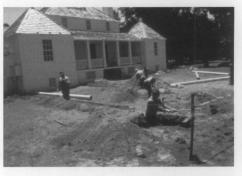
C. Develop new drainage systems for roof run-off that remove moisture from the base of the building. Photo: WPTC, NPS.
