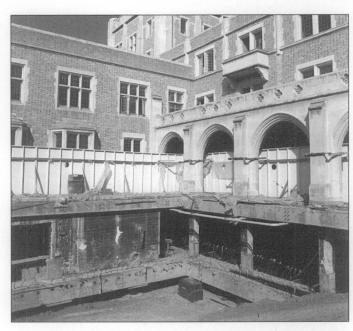
8. Full seismic restructuring to ensure that buildings survive a major earthquake with a minimum of damage may involve extensive reinforcement. Upon completion, the changes to this ca. 1932 Gothic Revival building to add base isolation at the foundation were not visually apparent. Photo: © Jonathan Farrer, courtesy University of California at Los Angeles (UCLA), Capital Programs.
