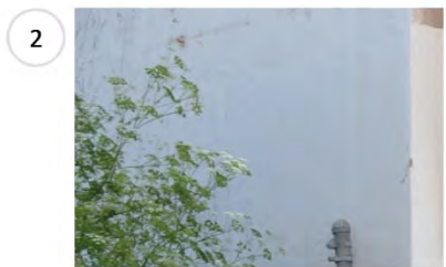
Painted stucco on concrete exterior walls
