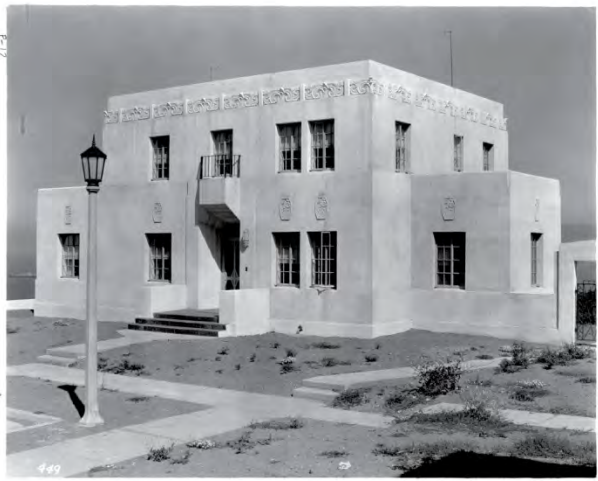
View of Building 11 looking north, c. 1934 . Note the original steel windows and the unpainted terra cotta features. (Courtesy of SFVAMC)
