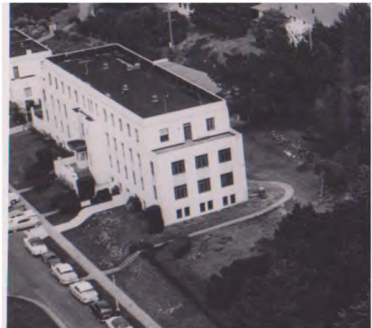
View of Building 8 looking north, c. 1950 . Note the original steel windows, unpainted terra cotta spandrels, and lack of 3rd floor additions on each stepped side wing. (Courtesy of SFVAMC)
