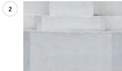
Painted stucco on concrete exterior walls
