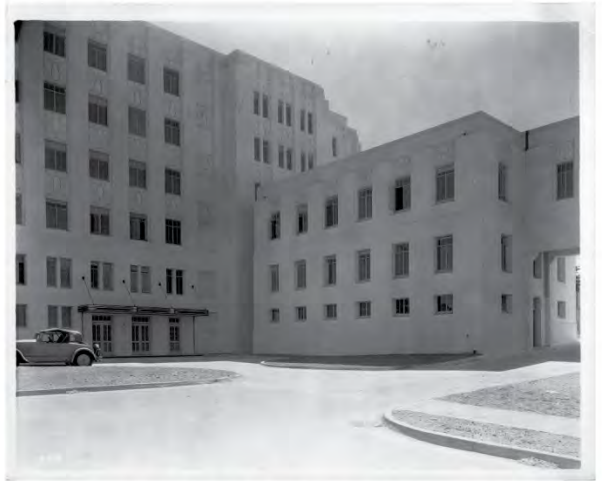
View of Building 4, c. 1934 . Note the original steel casement windows and the unpainted terra cotta spandrels. (Courtesy of SFVAMC)
