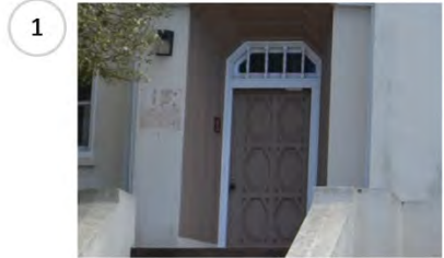
Original decorative wood doors and transoms; stepped concrete arches at door surround
