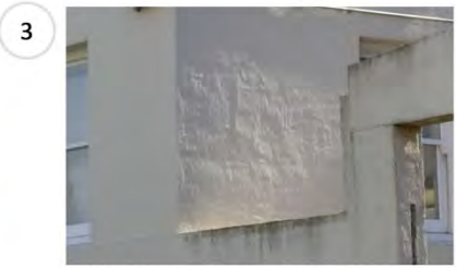
Painted stucco on concrete exterior walls
