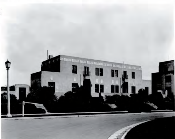
View of Building 9 looking east, c. 1934. Note the original steel windows and the unpainted terra cotta spandrels. (Courtesy of SFVAMC)
