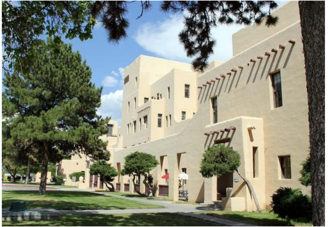
New Mexico VA Health Care System (NMVAHCS)
