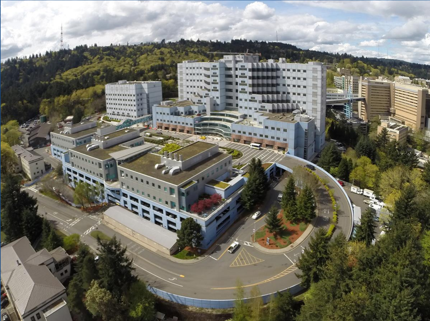
VA Portland campus aerial view
