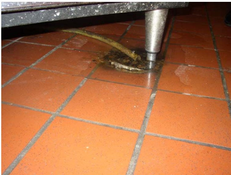
Picture 4 – Canteen Floor Drain
