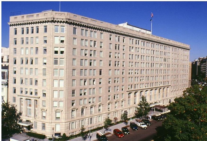
Figure 1. Veterans Affairs Building, Washington, DC. (Source: https://www.gsa.gov/ , accessed June 24, 2021).
